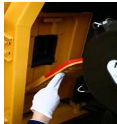
Replace A/C filter
