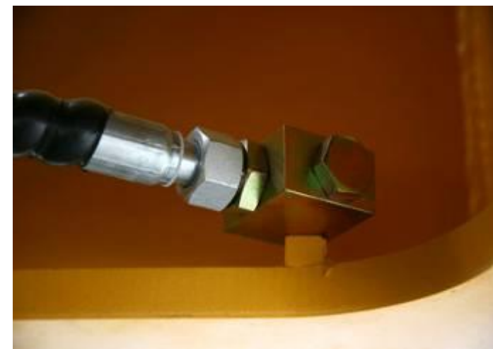
Swing motor oil drain
